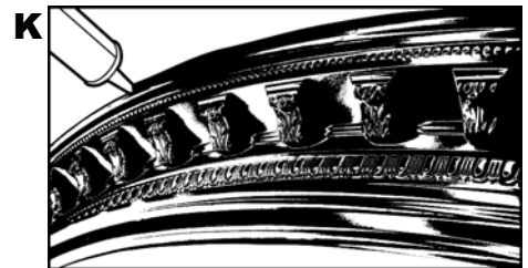
Apply paintable caulk to edges
