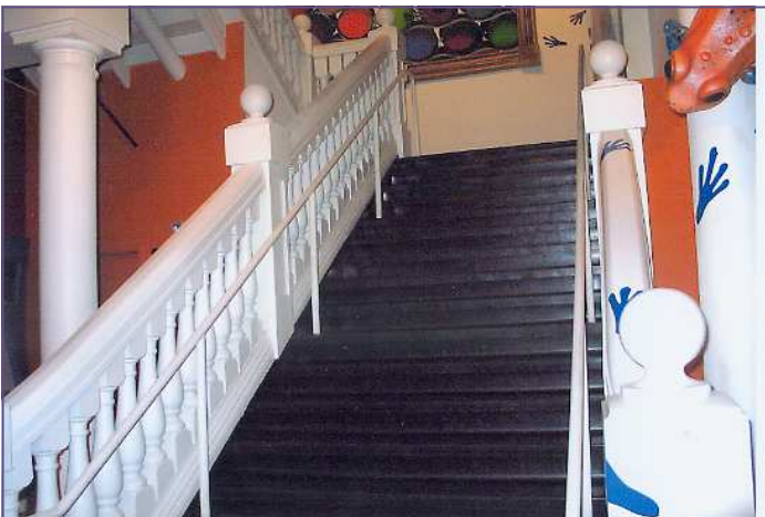
Left: Adding another element of challenge is the slight radius at the bottom of the stair run.
