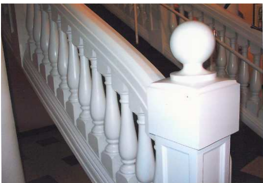
Left: Adding another element of challenge is the slight radius at the bottom of the stair run.
